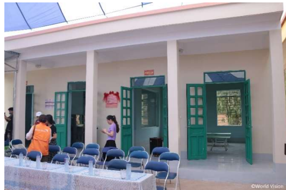
The new kitchen facility in the kindergarten
