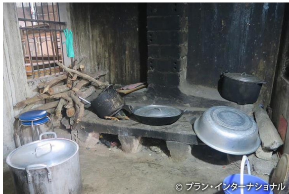
The Current Cooking Facilities at the Elementary School
